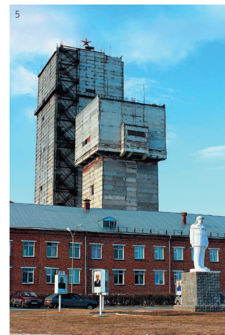
5. Severopeschanskaya mine: central group of pits with tower type headworks.
