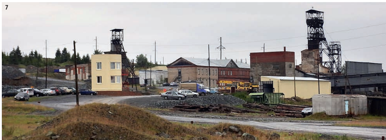
7. Mine headworks at the Saranovskoe deposit.
